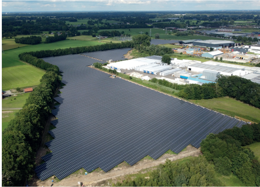
Hof van Twente PV plant into operation (credit: BELECTRIC)
